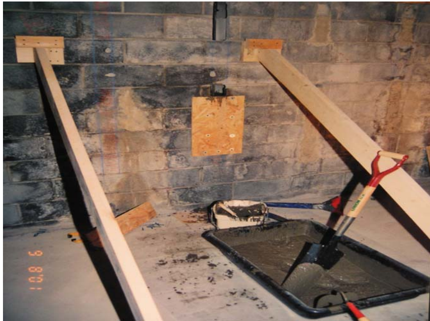
Figure 10 Slots covered and cores filled with relatively fluid concrete mix.
