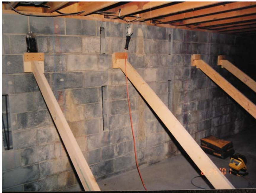
Figure 8 Slots cut for access into cores of block.
