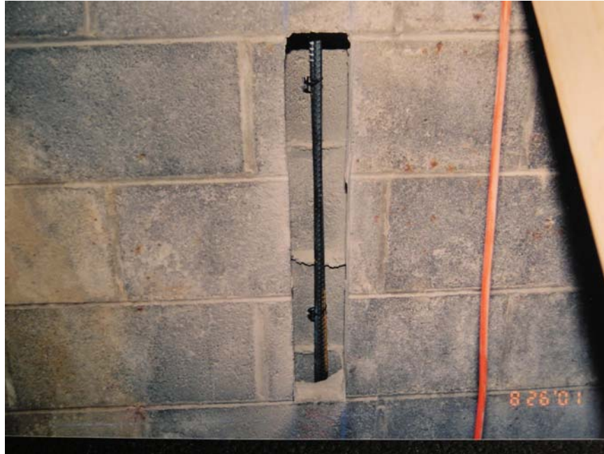
Figure 9 Steel reinforcing rods set in core. Note location and long lap.
