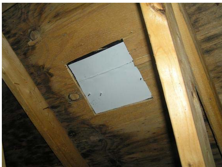
Figure 11 Roof deck clear of mold growth at roof vent.
